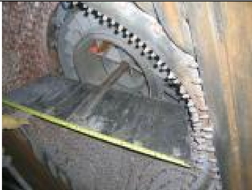
Figure 6: Steel form to properly contour burner throat. This gives the proper shape to the burner throat for efficient burner operation
