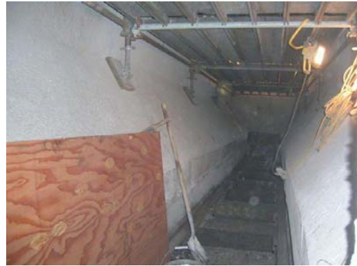
Figure 11: Completed ash hopper installation
