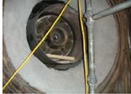
Figure 15: Completed burner throat
