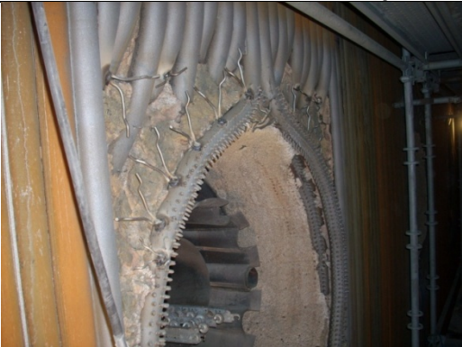
Figure 6: Steel form to properly contour burner throat. This gives the proper shape to the burner throat for efficient burner operation
