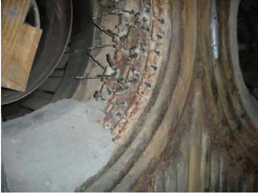
Figure 14: Thermbond Formula 15R partially installed in burner throat
