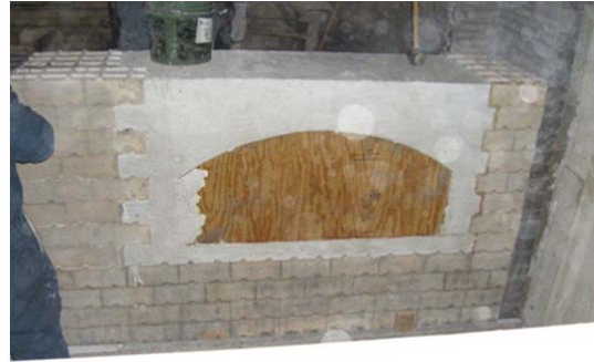
Fig. 11. No. 2 Archway Installation
