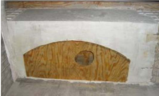
Fig. 10. No.1 Archway Installation
