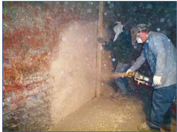
Figure 5. Incinerator side wall, gunning overlay.
