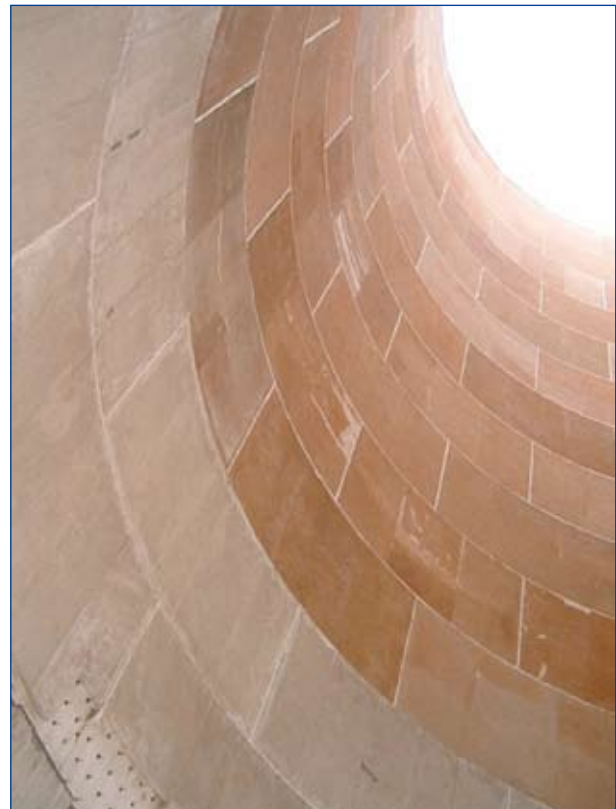
Figure 2. Completed ground flare.
