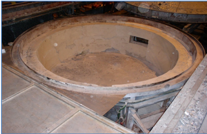
Fig. 5 Aluminum round top melting furnace veneer lined with LPB refractory materials
