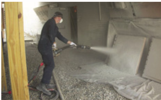
Thermbond gunning demonstration presented by Jens Decker, Vice President of Engineering
