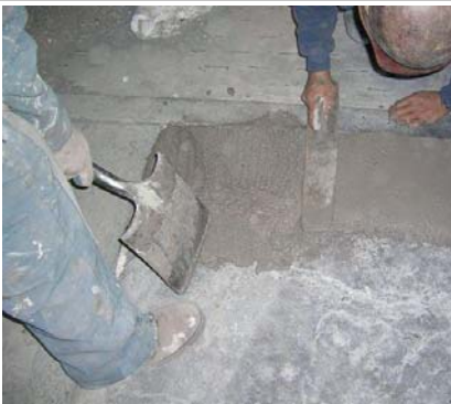
Placing of Phoscrete 602-L
