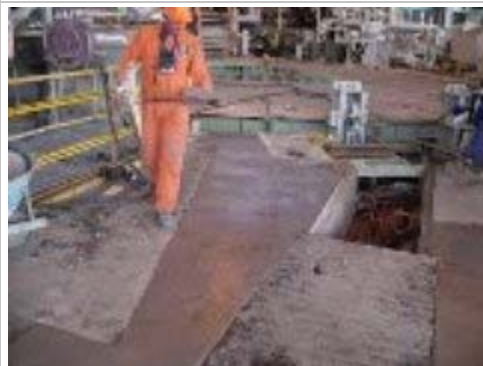
Completed area of Phoscrete 602 repair.
