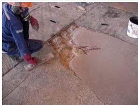
Waiting for final pour in the area to be repaired.
