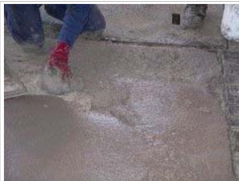
Installing Phoscrete as an overlay on existing concrete.
