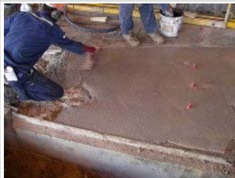
Installer finishing surface as Phoscrete material is poured.
